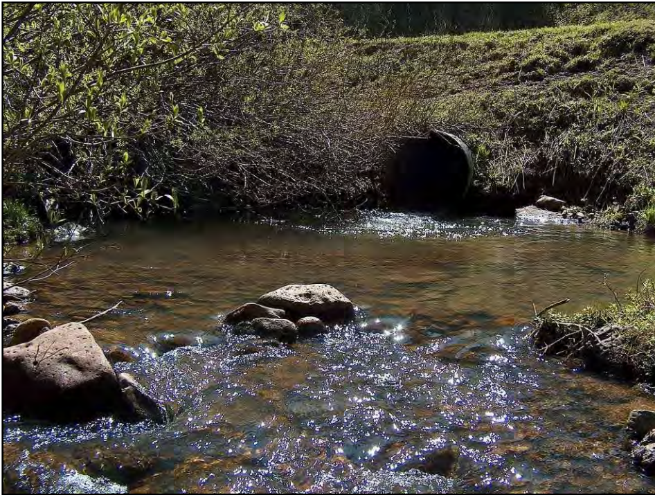
Figure H.2b. North Thompson Creek Culvert Outlet.
