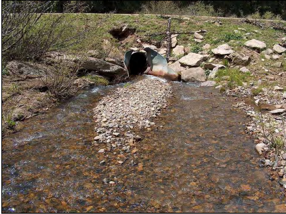
Figure H.2a. North Thompson Creek Culvert Inlet.
