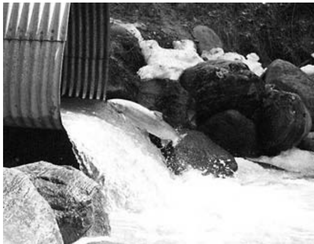
Figure 2.3. Drop and Velocity Barrier.
