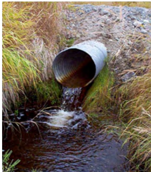
Figure 2.2. Perched Outlet, Leap Barrier.
