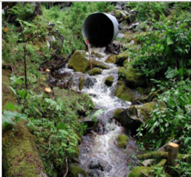
Figure I.1. Tributary to Bear Creek Culvert Outlet.
